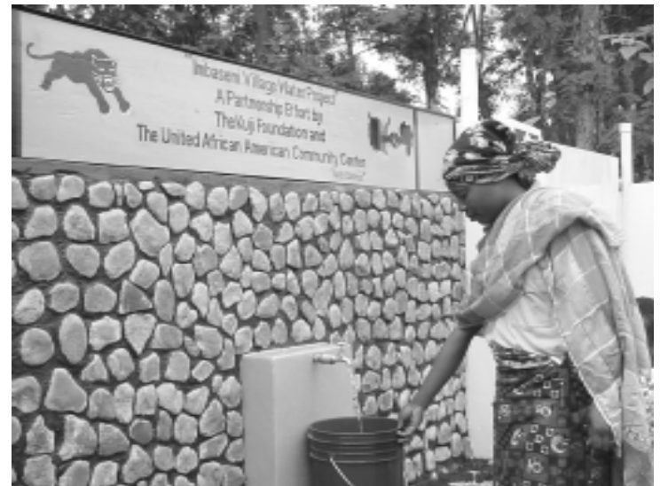
A villager uses the new faucet.
